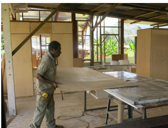
Carpenter busy at work at Kompiam District Hospital
