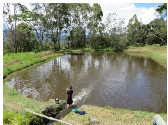
Hydro Water Scheme Telefomin
