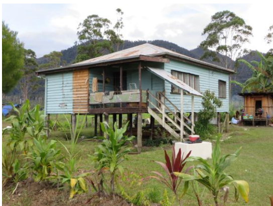
Staff Housing at Telefomin Hospital
