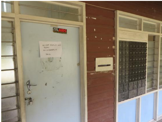
District Health Office in Telefomin
